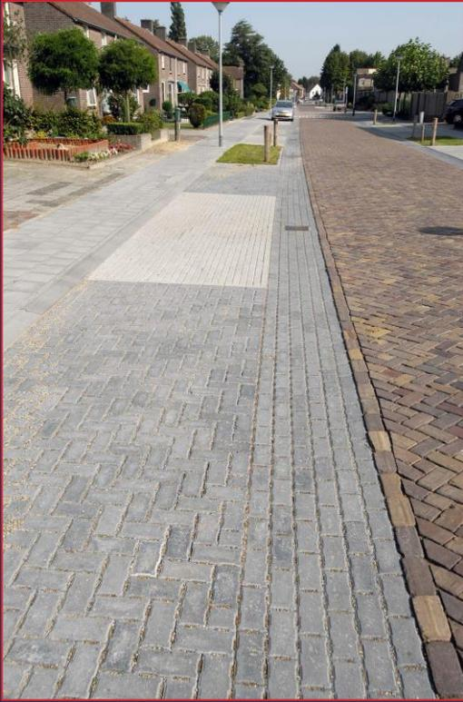
The Kellen H2O paving system is an innovative permeable block paver that provides an attractive, durable surface finish, while also acting as an effective drainage solution. Available in Breccia and Lavarò finishes and corresponding colours.
