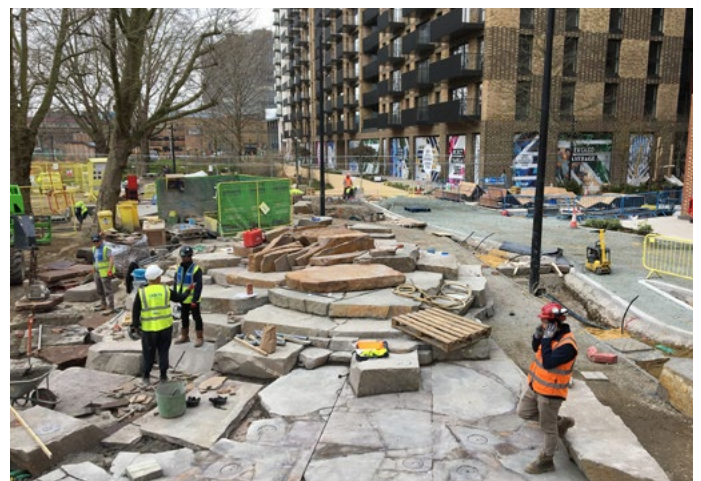
Construction of Elephant Springs - March 2021
