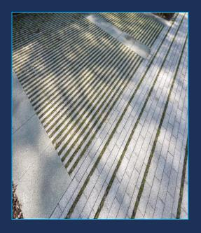
Hydro Lineo includes three different models of concrete pavers. These three models have a uniform nominal outer size. The width of the widened joint is the only variation per model. The three different models can therefore be used individually as well as being mutually exchangeable. Thanks to the increasing width of the widened joint, the street scene shows Hydro Lineo in a smooth transition from a closed to an open pavement, and back again.
