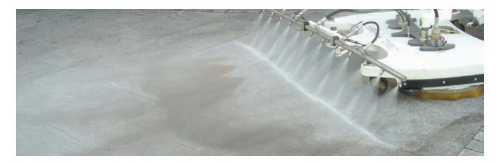
staining. To remove rust stains, the surface should be wetted and the affected area treated with a prop solution. After cleaning, the paving should be well washed down to remove all traces of the acid.
